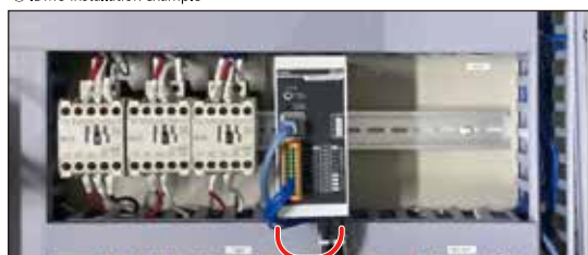
◎ IDMU installation example
